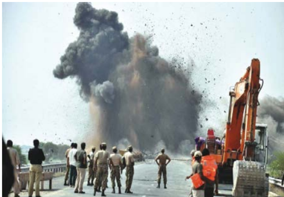
Breaching Section activated at Head Muhammad Wala Bridge (Multan)
